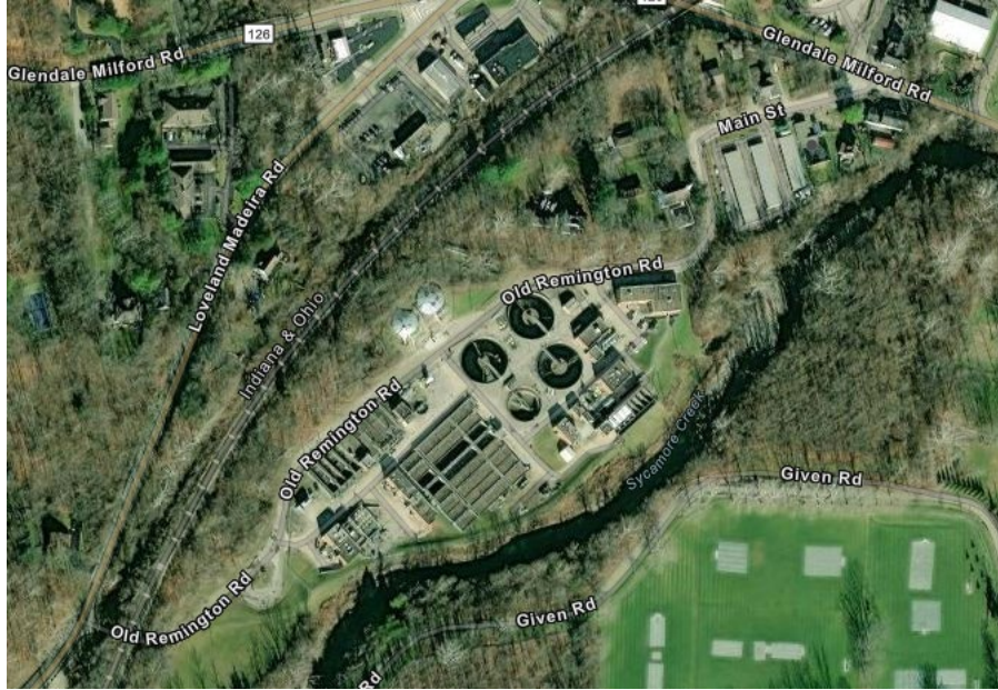
Figure 2. Sycamore Creek Wastewater Treatment Plant
