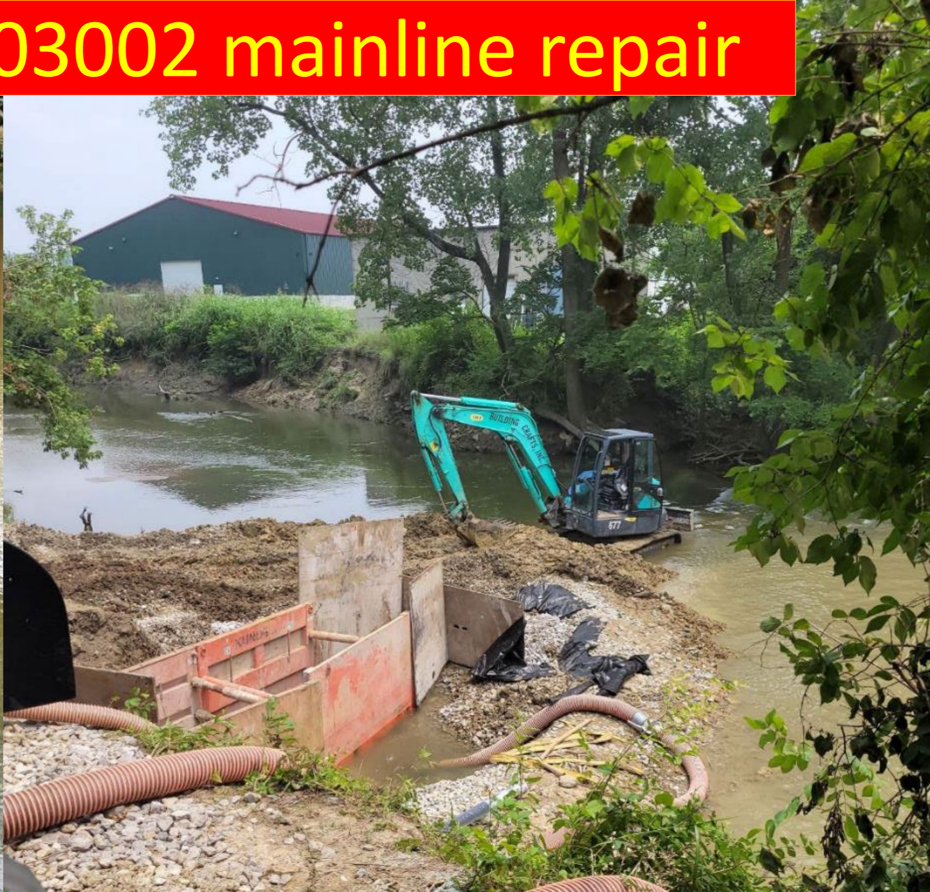
Original sewer encasement at creek crossing
